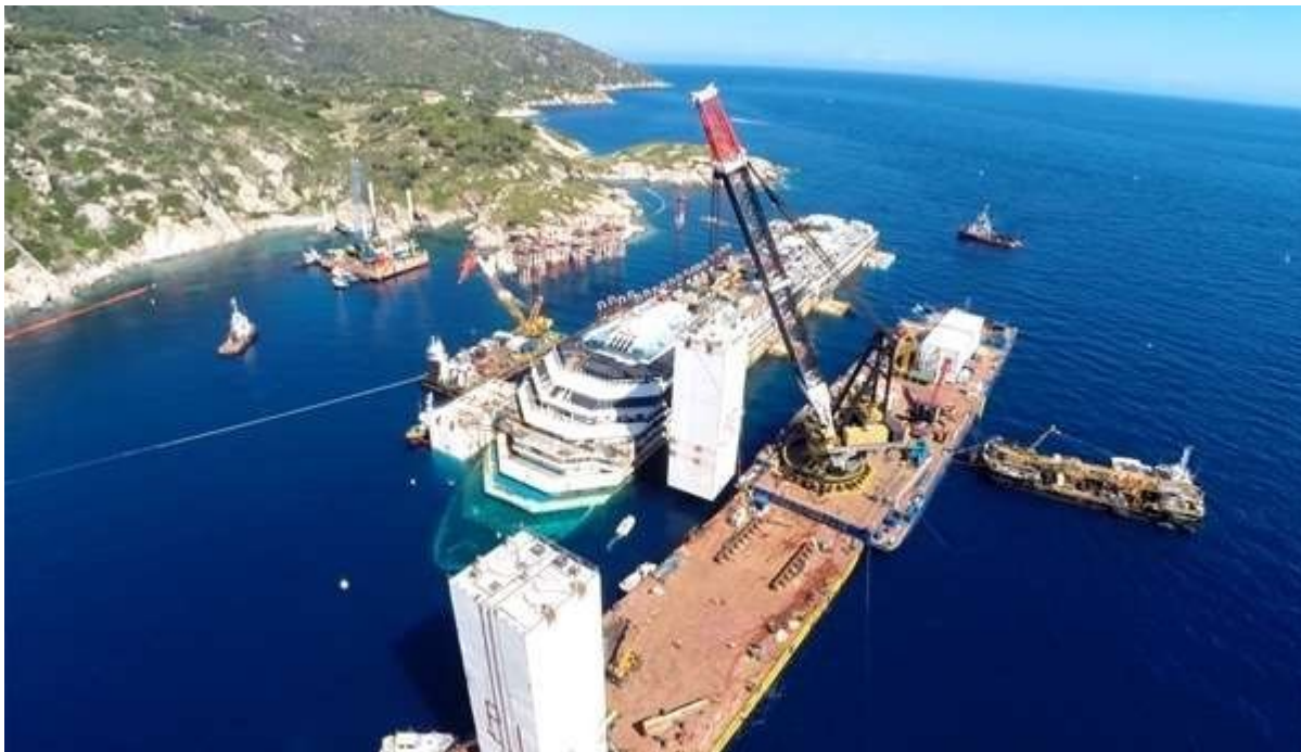
Installation of 850 ton buoyancy tanks on Costa Concordia, Italy 2014, using crane barge MB1.
